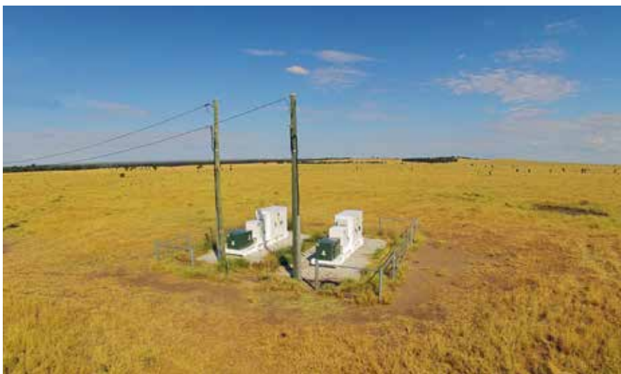
Our GUSS battery energy storage units, this one in Kinnoull, are both enhancing the local capacity of the network and managing voltage issues, for a lower cost than traditional network solutions
