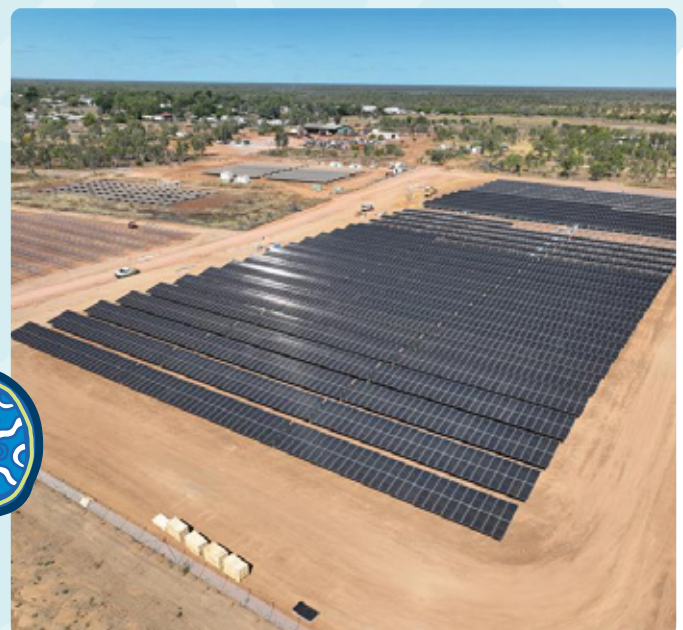
Below: Doomadgee Solar Farm
